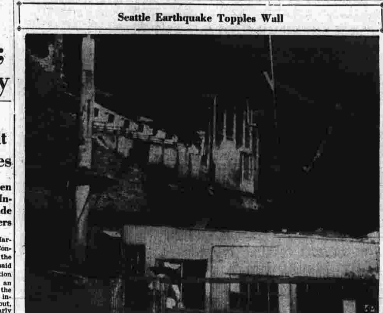
Seattle Earthquake Topples Wall
